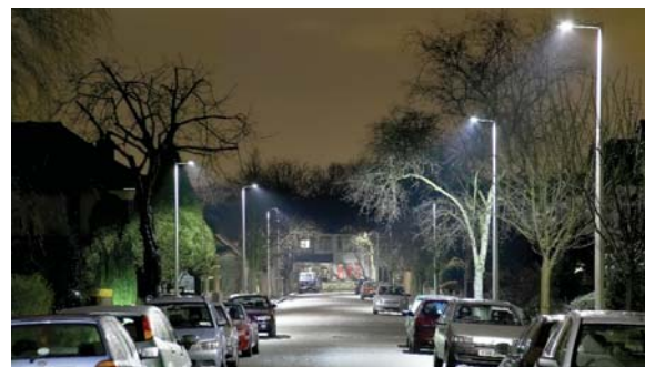
After - New technology London Borough of Redbridge
